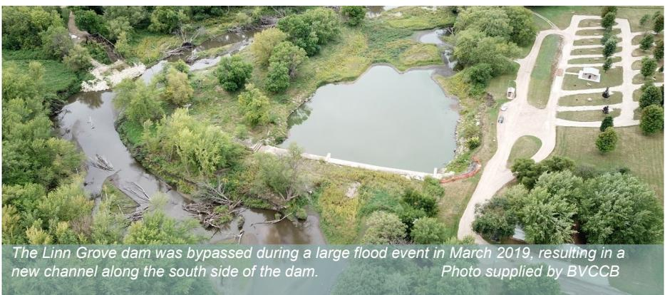
*The Linn Grove dam was bypassed during a large flood event in March 2019, resulting in a new channel along the south side of the dam. Photo supplied by BVCCB*
